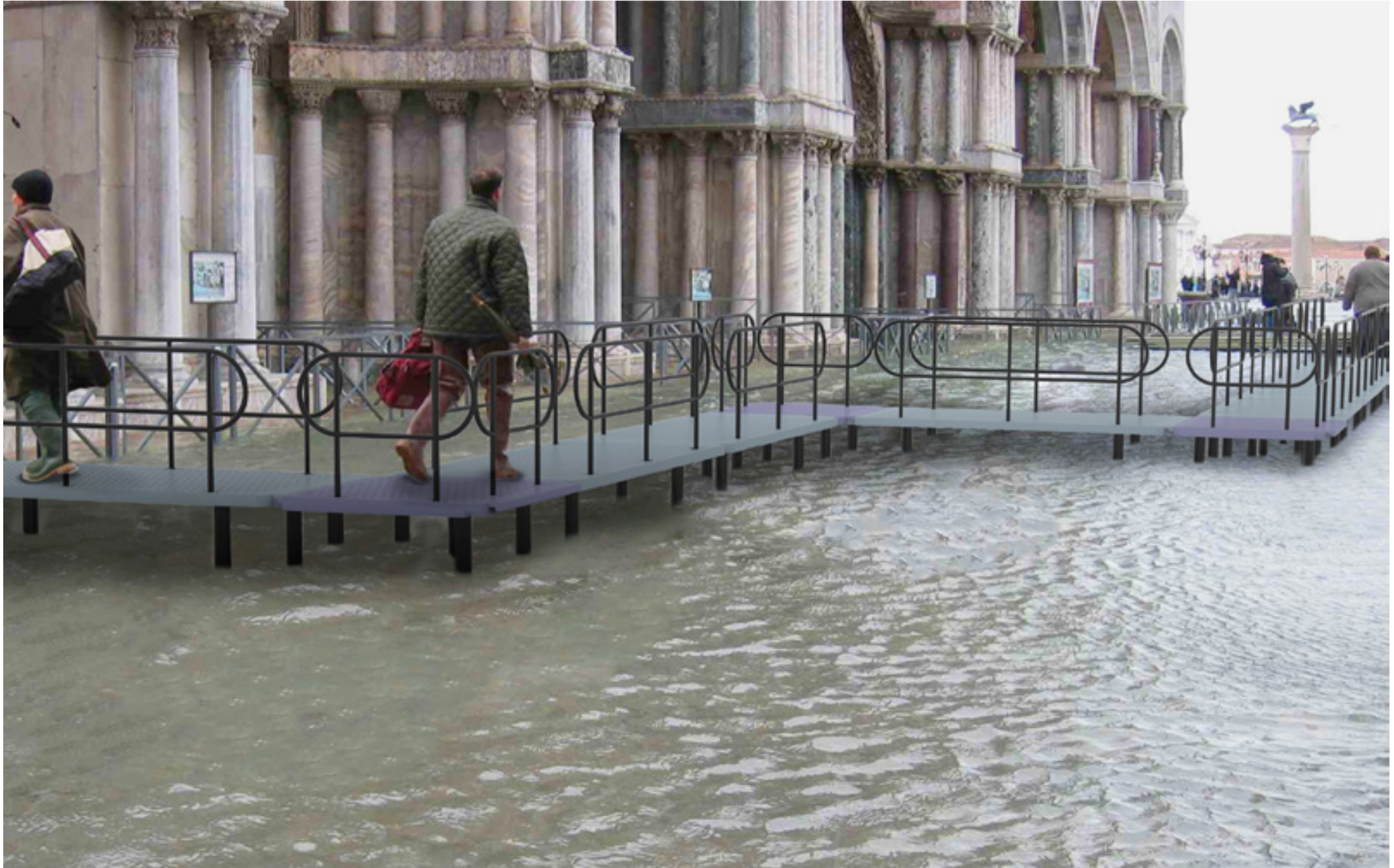
> The rotomoulded platforms are modular to form different routes to connect areas of the city, allowing people to move with high tide.
